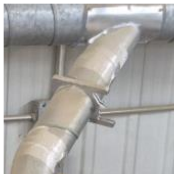
Figure 3-6 - Registre guillotine manquant
